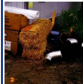
Halmballs on construction site
