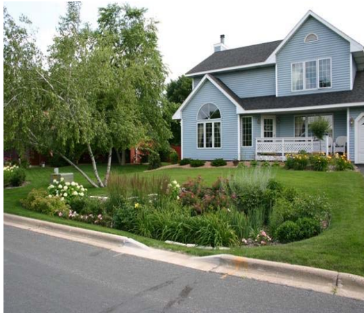
This Burnsville rain garden features a specially designed curb-cut that diverts and soaks up water from the street. (Photo courtesy Barr Engineering Co.)
