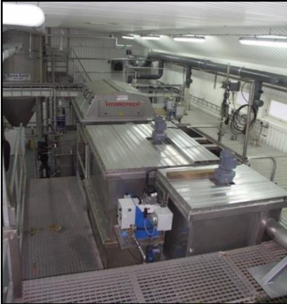
Drumfilter Installation in the Avesta WWTP, Sweden
